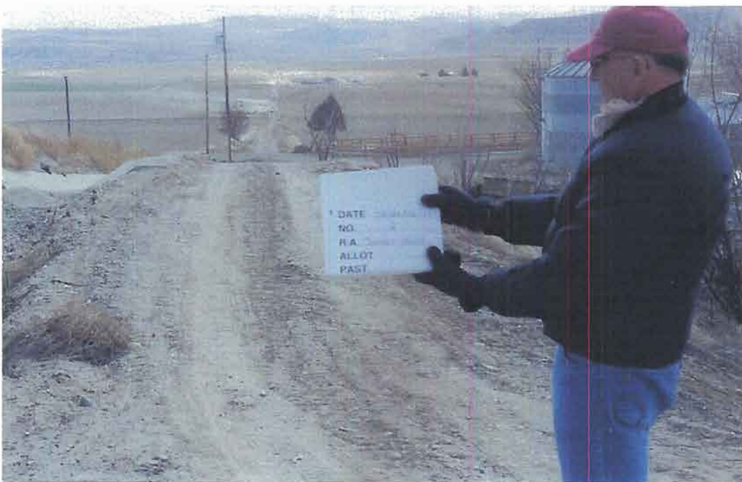
Sunset Valley Irrigation Enhancement Project Photopoint #2: Pipeline and Pivots – Phase I 2/28/02 (before)
